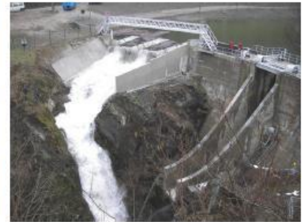
Goulours dam (France, 2006)
