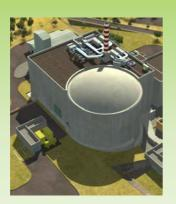
a fast-spectrum experimental system with a power range 50-100 MWth to support development and demonstration of innovative reactor-cooling technology (Gas/lead)
