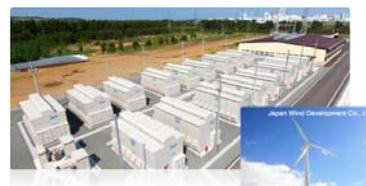
34 MW NAS alongside 51 MW Wind Farm (Futamata, Japan)
