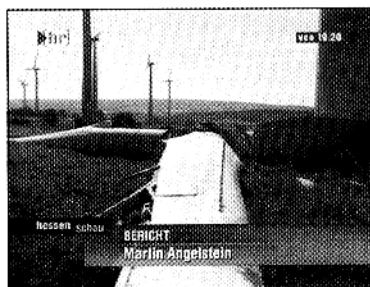
Sept. 9, 2002: Rotor severed NEG-Micon M 1500, year of construction: 1996 'Hoher Vogelsberg' wind farm, Location: Ellrichstein, Hildesheim
